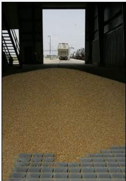
Trucks back up to a bay, where they dump their corn onto grates.
